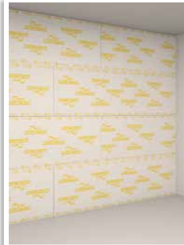
2. Boards installed horizontally
